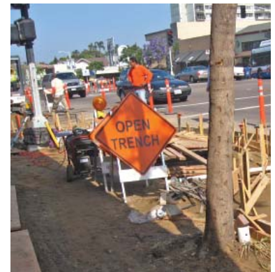
Washington and Goldfinch south-east curb under construction.
