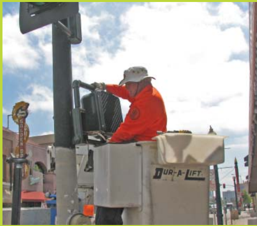
City Transportation crew at Fourth and University installing new pedestrian signals.
